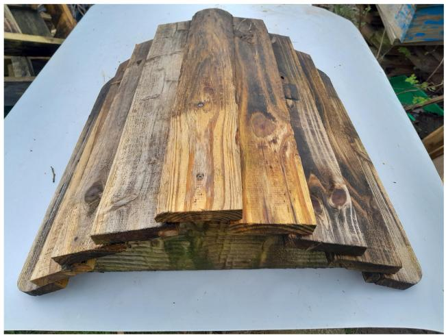
roof is complete with slats glued and screwed into place.
