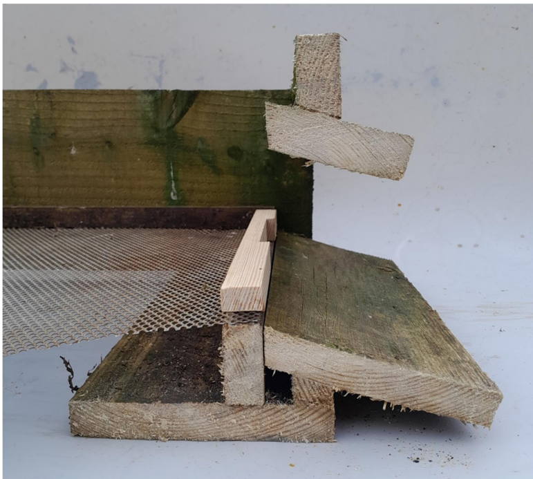
Cross-sectional view of the front of the WBC base and landing board. National floor and entrance cross-section is also shown in situ.
